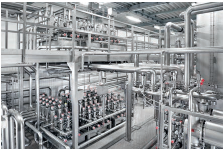
Two-level, fully-automatic valve manifolds with DN125/100 mixproof double seat valves, to connect ten tanks to seven filling lines.
